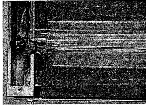
2. Loosen the screws on the heat tube collars (one on each end of the tube).
